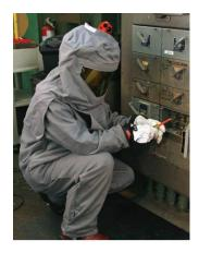
Arc Flash Boundaries and potential incident energies are calculated during an Arc Flash Hazard Analysis and are used to alert workers of the dangers of working on energized electrical equipment. Arc Flash hazards are required to be labeled. An Arc Flash Hazard Analysis is
